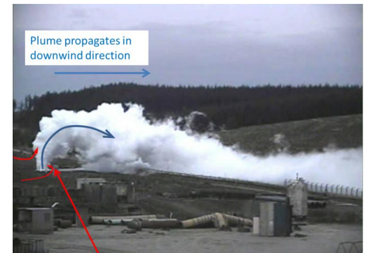
Fresh air entrainment possible around plume base
